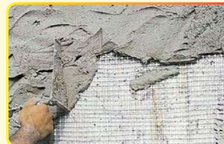
APPLICATION (PLASTER MESH)
